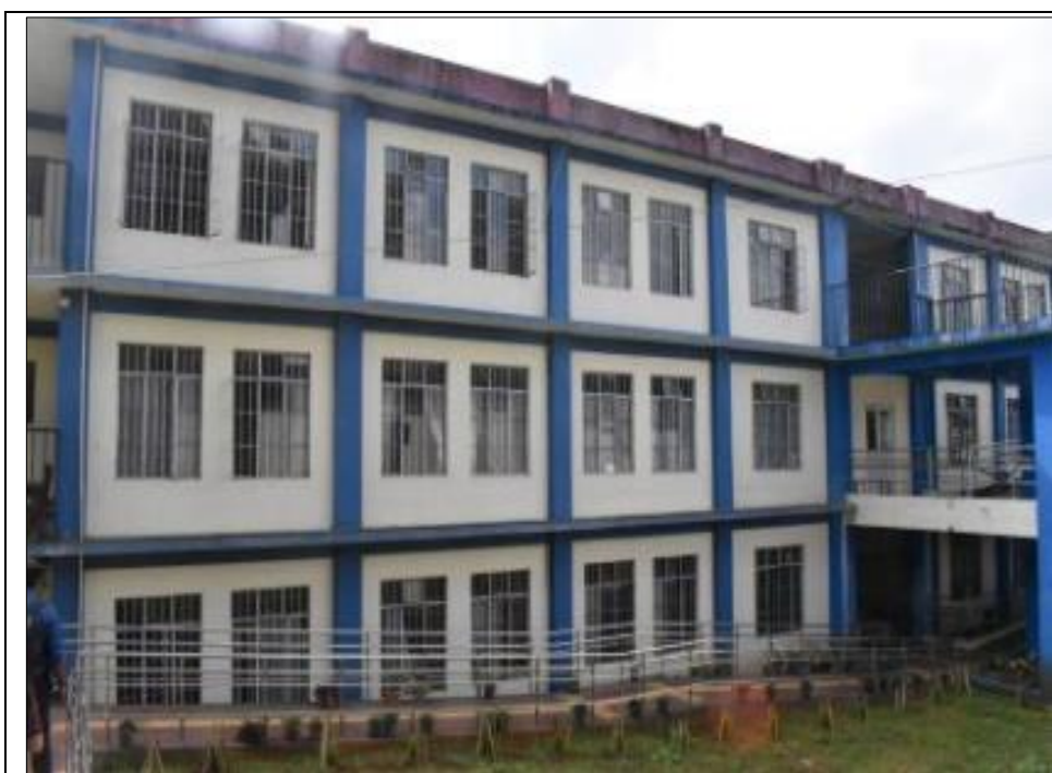
Figure 5: Photographic Exhibit of Shillong Pine Mount School
